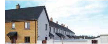
Social Housing Installation Co. Louth, Ireland
